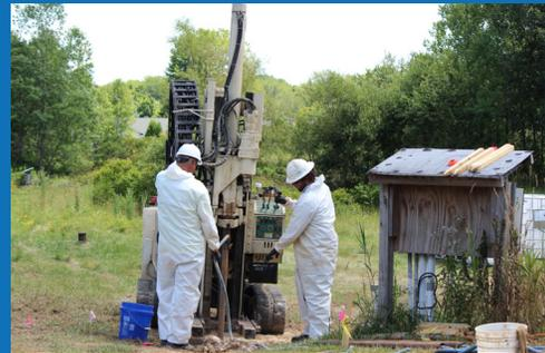
Cascade Technical Services crews provide calculated injections to remediate soil and groundwater contamination
