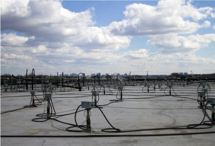
Did you know that thermal remediation is a powerful technology to clean up source zones at contaminated sites? That was confirmed recently when a client with a large Thermal Conduction Heating (TCH) site in NJ said that 10 months of thermal operations saved their client approximately 40 years' worth of existing pump and treat, with a potential cost savings of \$40M. What other technology can achieve that?
