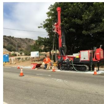
An air-vac unit was used to expose and mark an inactive water line, a process known as daylighting. Once the site was clear for drilling, the crew used a mini sonic rig to drill a pilot borehole. The lithology information gathered in that core sample was critical in designing the injection well specifications. A dual rotary drill rig was required to successfully place the 168 feet average depth, 14-inch diameter wells.
