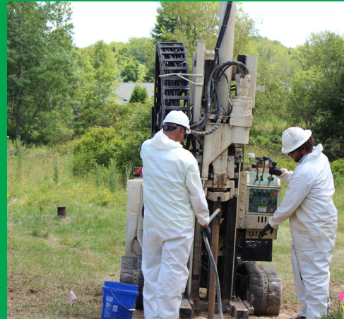
Cascade Remediation Services crews provide calculated injections to remediate soil and groundwater contamination.
